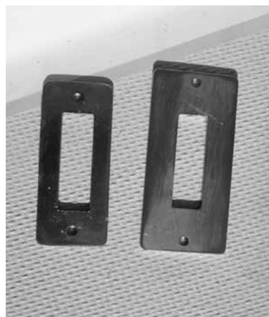
After I finished the project and stood there admiring my work I was hit with a "Homer Simpson" moment! Doooooh! I should have done what Don Casey suggests, over drill the holes, fill them with epoxy and then drill new holes for the cover plate screws into the epoxy. This will eliminate any water getting into the core.
