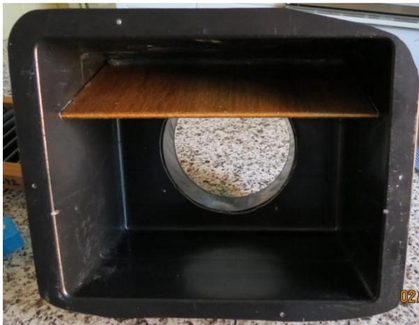
The baffle was made from a scrap piece of plywood and varnished, then glued in-place to meet the edge of the grill.
